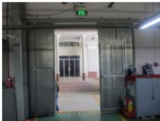
Emergency exit door.JPG
