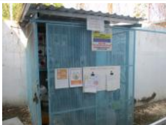
Chemical warehouse with safety signs.JPG
